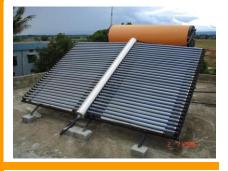
Solar Vacuum Glass Tube Water Heater is scientifically designed system to suit tropical, as well as high altitude sub zero regions. These systems are suitable for hard and saline water and are used for domestic as well as industrial application such as hotels, hospitals, dairies, hostels, nursing homes, feed water for boilers, process industries etc.
